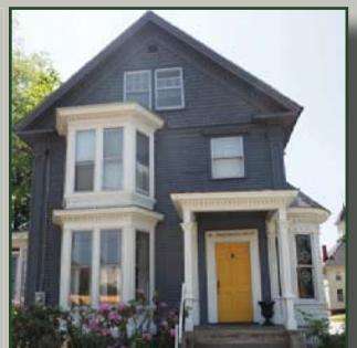
Gable roof and almost flat secondary roof forms.
