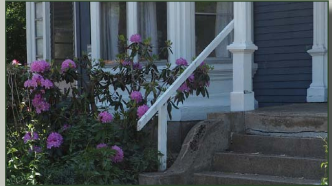
A simple painted wood handrail on the outside of the stoop does not detract from the design or damage historic material.
