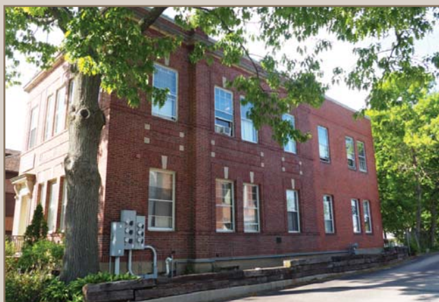
A subtle material color change and eliminating brick details differentiate between the historic building and the rear addition.
