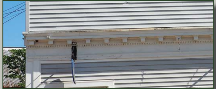
Match wood siding and decorative features when replacement is necessary.
