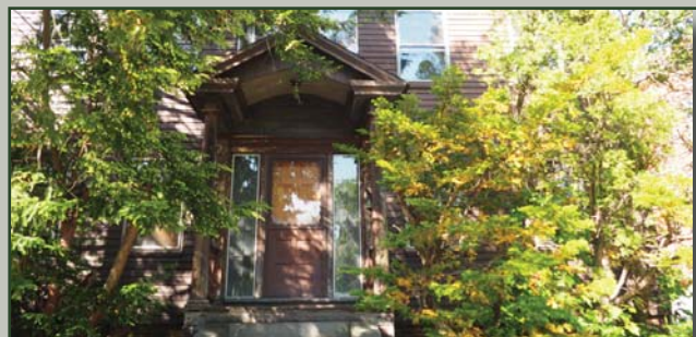
Large trees and bushes can hold moisture against wood siding which encourages rot.
