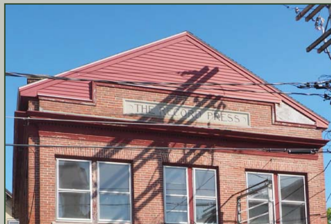
A gable roof was presumably added atop the parapet of a flat roof commercial building.
