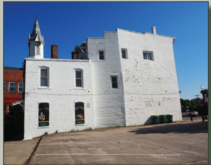
At bottom left the ground floor windows were bricked in and painted black which creatively maintains the visual repetition of "windows" on this facade.
