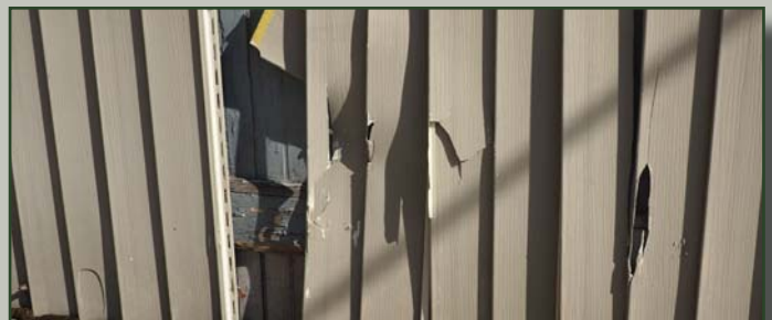
Remove vinyl siding to reveal the original wood material as shown here.
