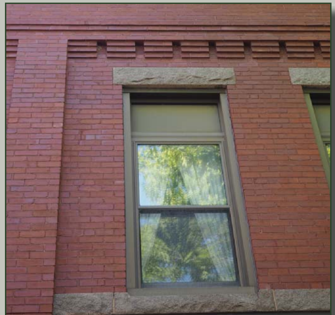
A smaller window frame was fit into a large historic window opening creating a gap at the top that was filled in with painted wood.
