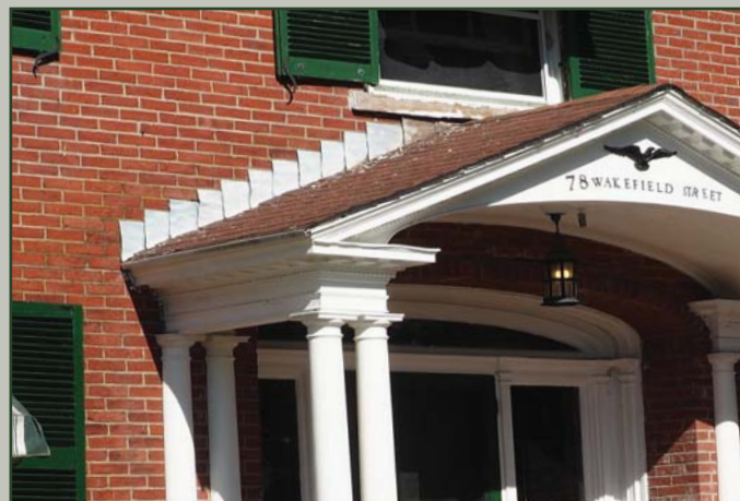
Flashing detail at the porch roof stands out against the brick facade, but is important waterproofing.
