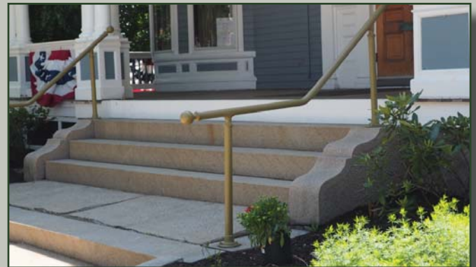
A simple metal handrail is an appropriate solution.
