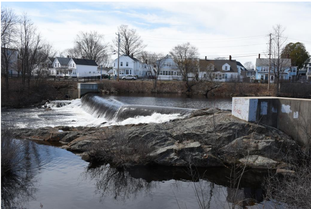
Photo 70) Upper Dam, Cocheco River at Bridge Street, looking west
