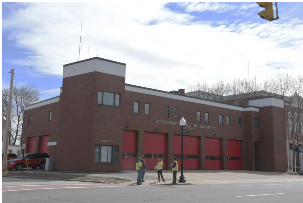
Photo 14) 37 Wakefield Street, Rochester Fire Department, looking southeast
