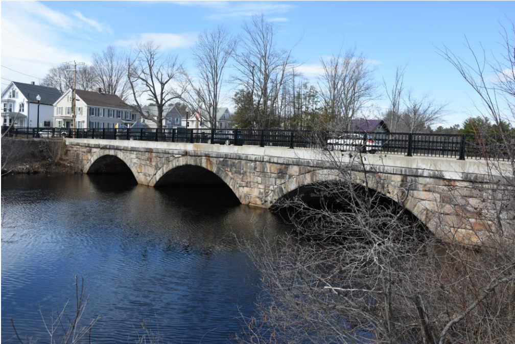
Photo 58) North Main Street Bridge, looking northwest
