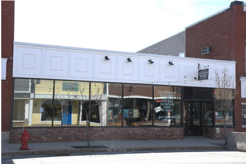
Photo 40) 32 North Main Street, looking southwest
