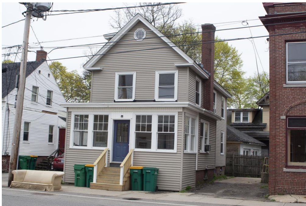
Photo 112) 113 Portland Street, looking south
