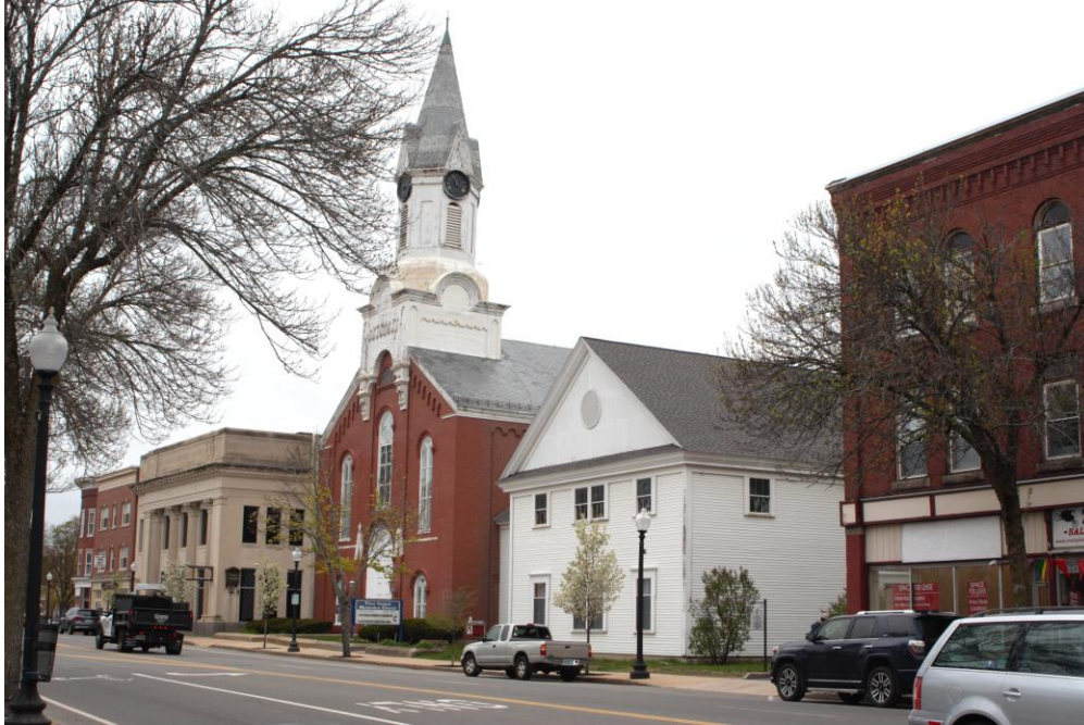
Streetscape of South Main Street, northeast side, showing the United Methodist Church (Preservation Company)
