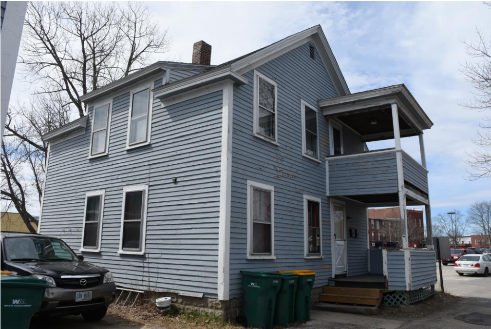
Photo 6) 18 Wakefield Street Rear, looking southwest
