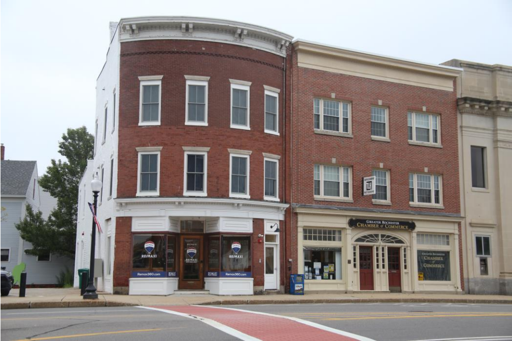
Photo 83) 10 (left) and 18 (right) South Main Street, looking east
