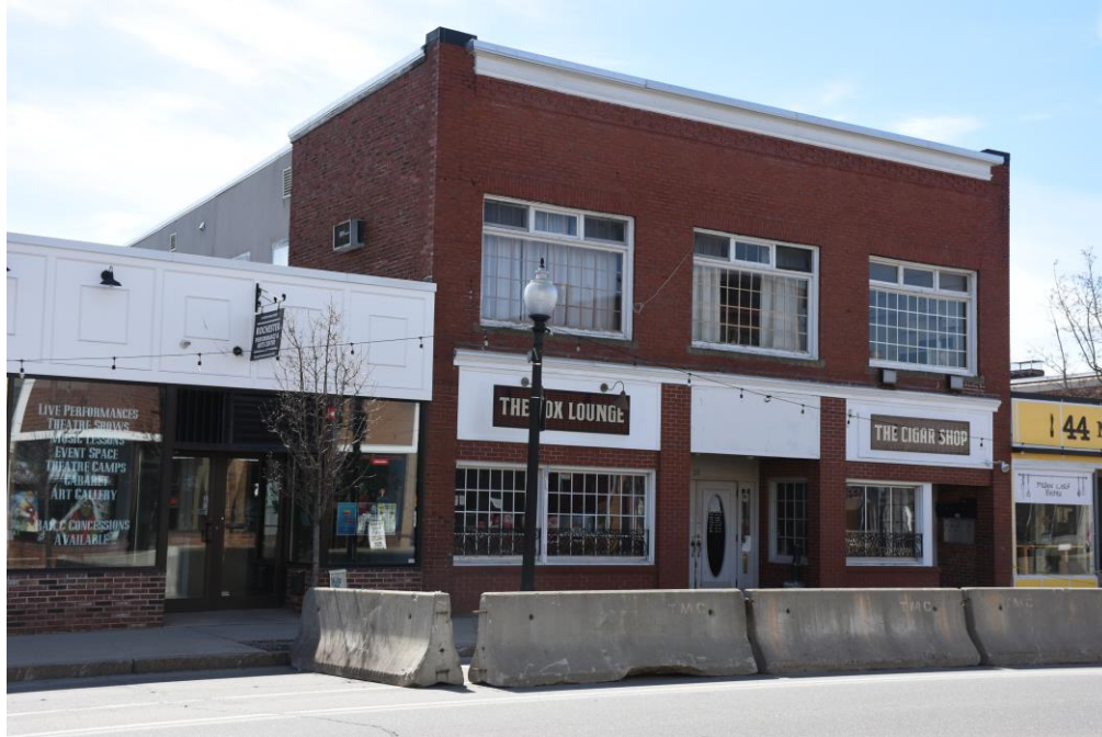
Photo 41) 38-44 North Main Street, looking southwest
