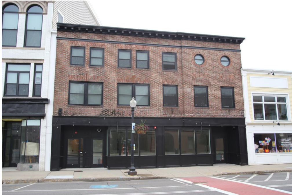
Photo 35) 12-14 North Main Street, looking southwest
