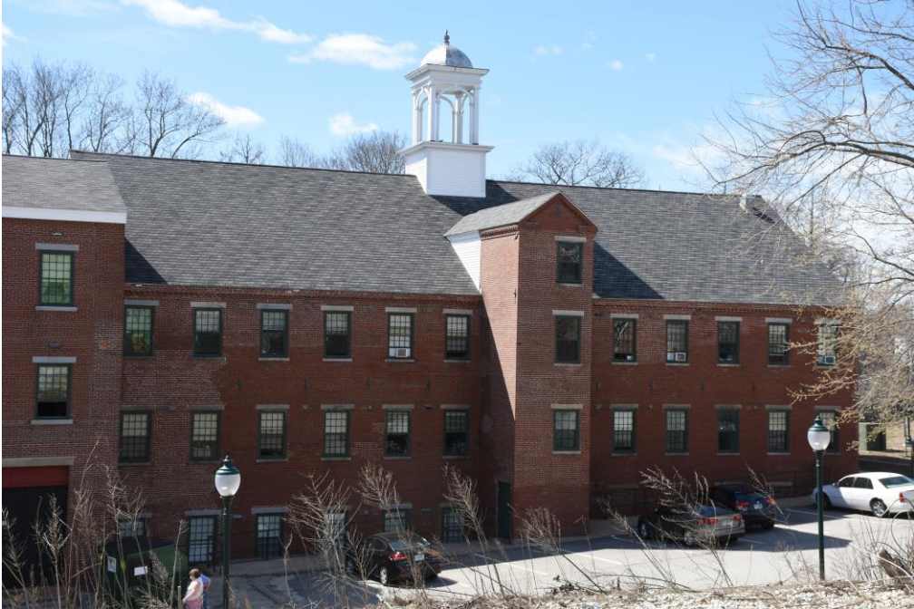
Photo 67) 6 Bridge Street, looking west
