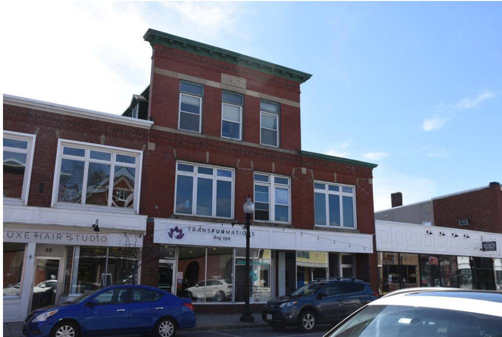
Photo 37) 26-28 North Main Street, looking southwest
