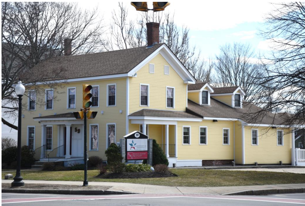
Photo 92) 59 South Main Street, looking south
