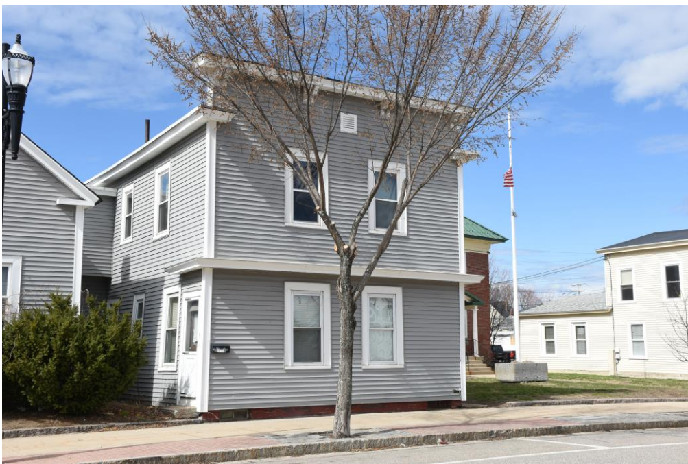
Photo 78) 52 Hanson Street, looking north
