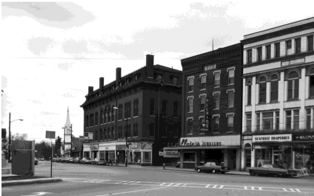
Central Square, looking southwest toward the McDuffee Block at left. (National Register District Nomination)
