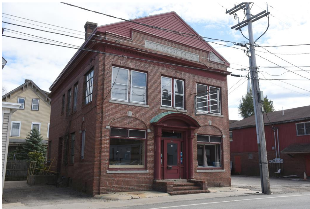
Photo 110) 109 Portland Street, looking south
