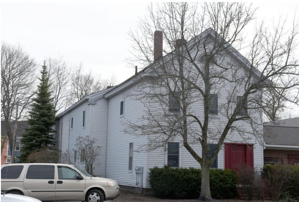
Photo 64) 21 Union Street, looking southeast
