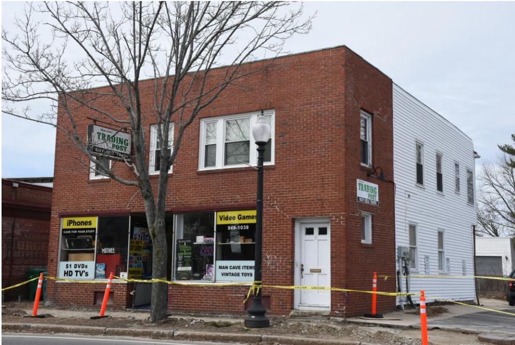
Photo 59) 4-6 Union Street, looking west
