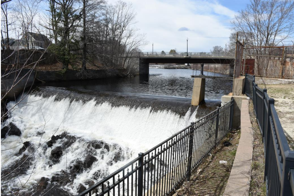
Photo 69) Lower Dam, Cocheco River at Bridge Street, looking northwest
