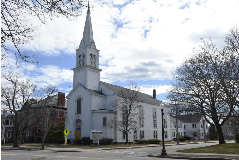
Photo 95) 63 South Main Street, looking south
