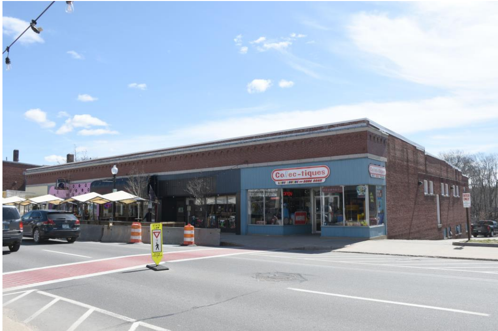
Photo 44) 48-56 North Main Street, looking southeast
