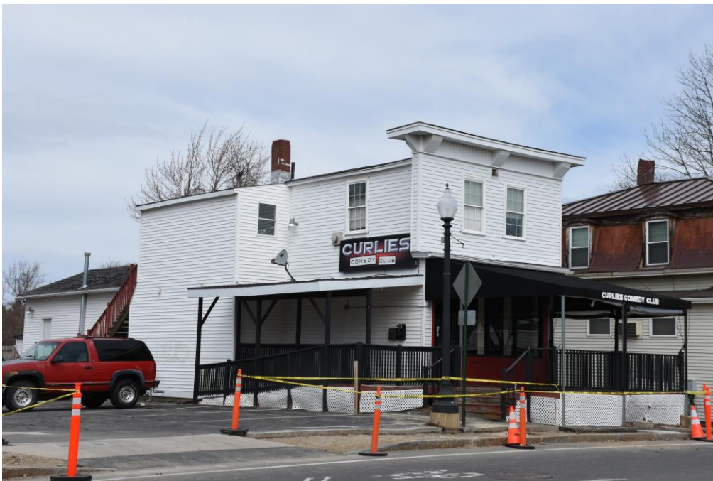
Photo 60) 12 Union Street, looking north
