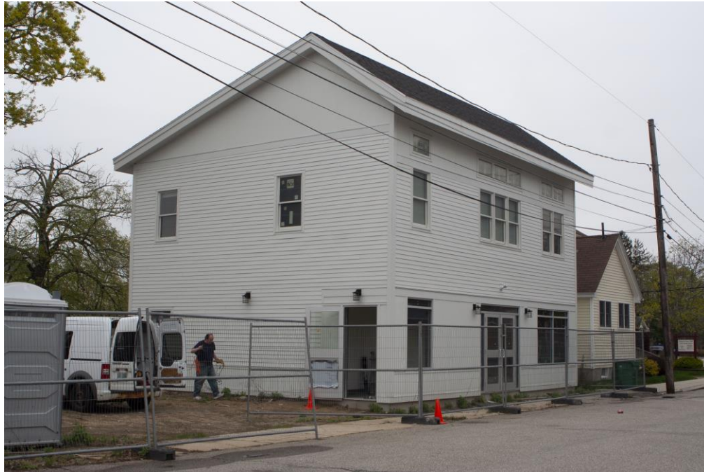
Photo 113) 5-7 Dreyer Way, looking south
