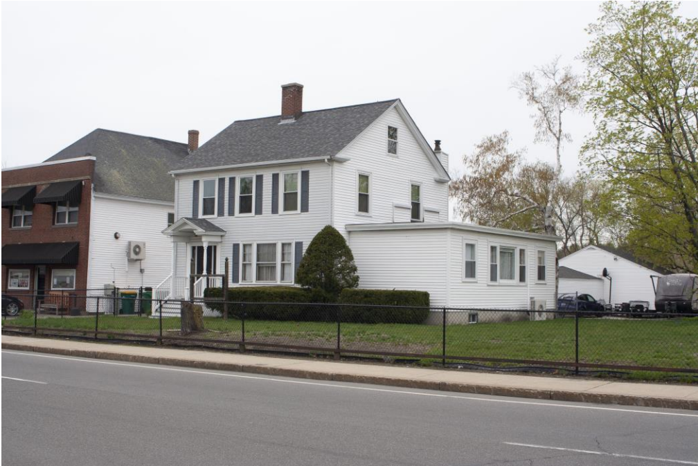
Photo 66) 24 Union Street, looking west
