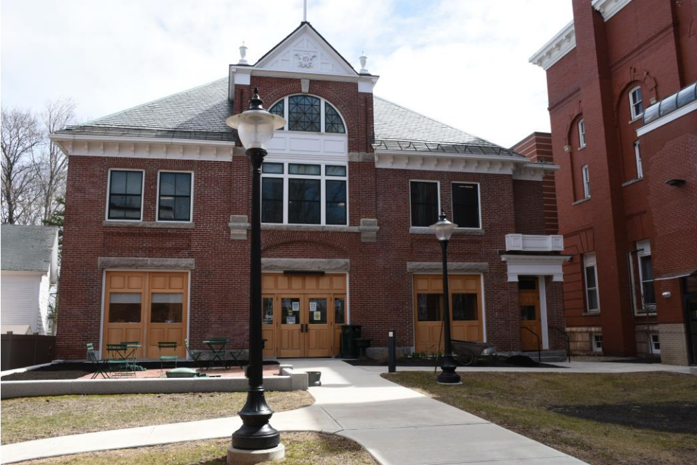
Photo 12) 33 Wakefield Street, City Hall Annex, looking east
