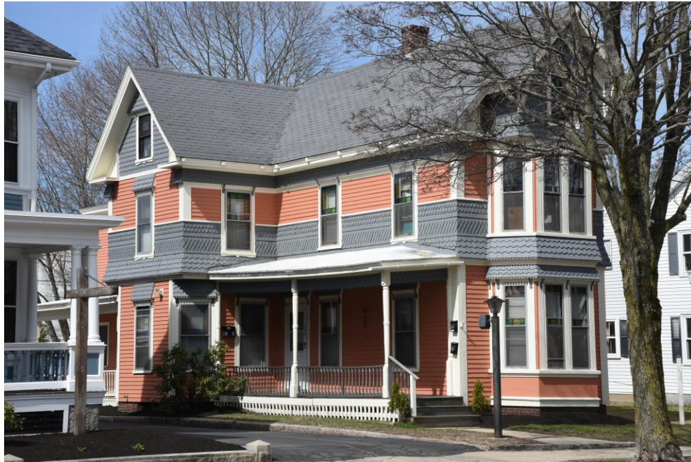
Photo 13) 36 Wakefield Street, looking northwest
