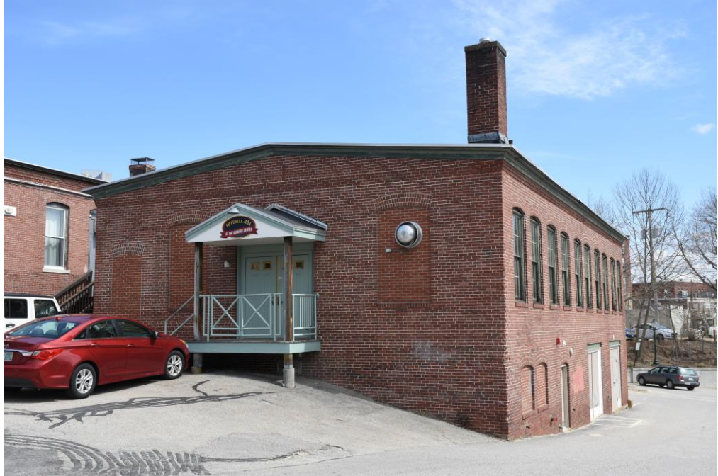
Photo 43) 48 North Main Street, looking east
