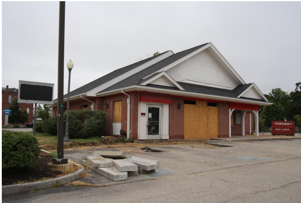
Photo 101) 77 South Main Street, looking south
