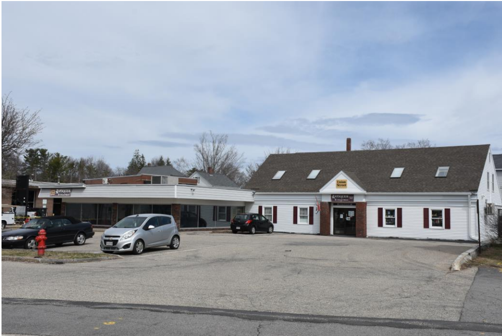
Photo 63) 19 Union Street, looking north
