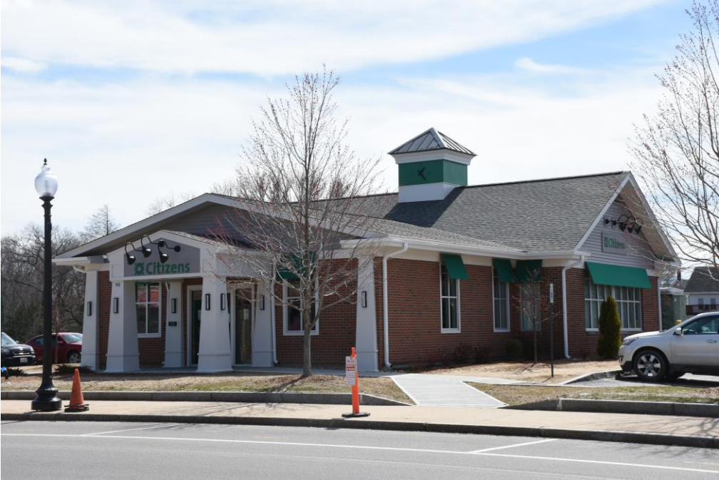
Photo 50) 90 North Main Street, looking south
