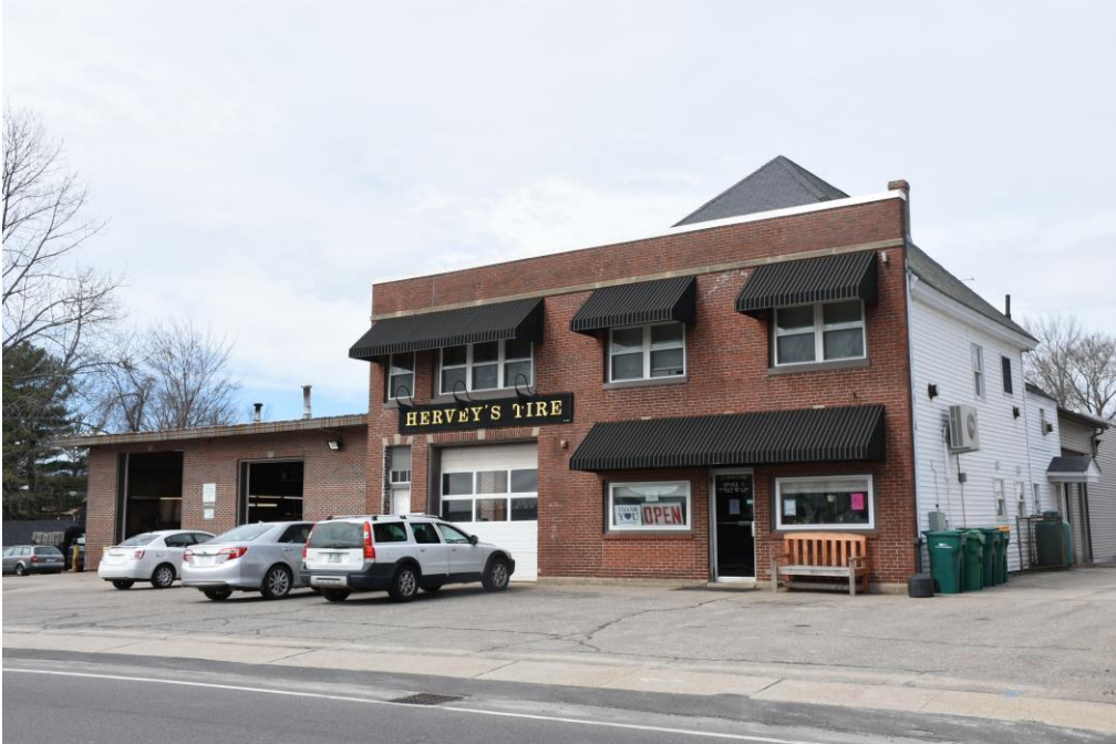
Photo 65) 22 Union Street, looking west
