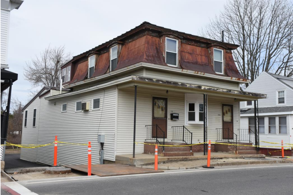
Photo 61) 14 Union Street, looking north
