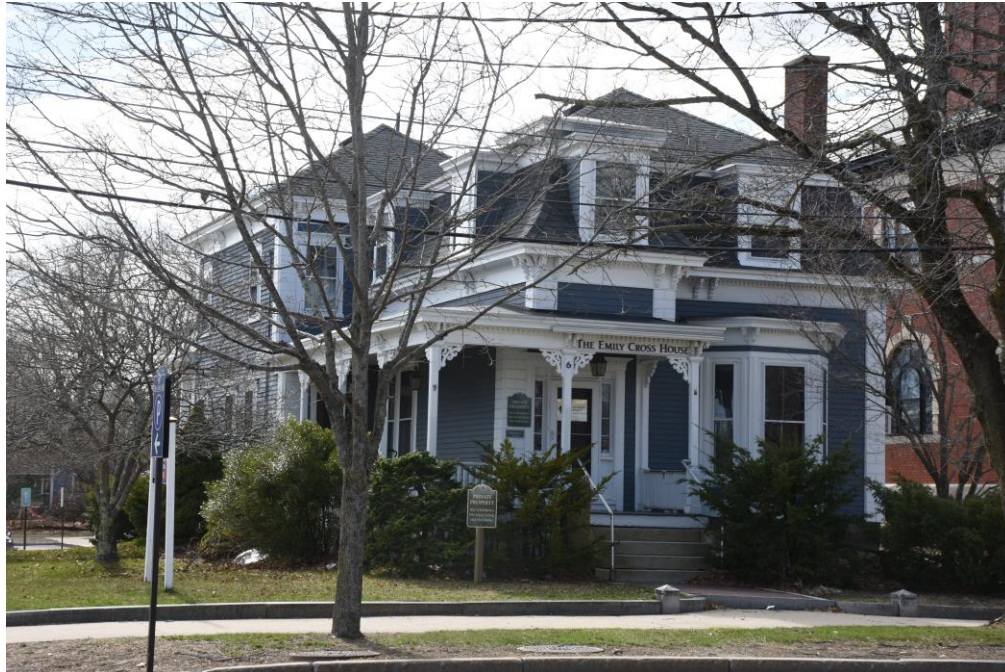
Photo 99) 69 South Main Street, looking west
