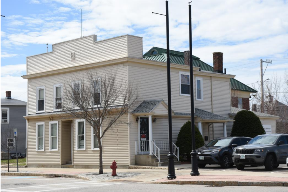
Photo 81) 60 Hanson Street, looking west
