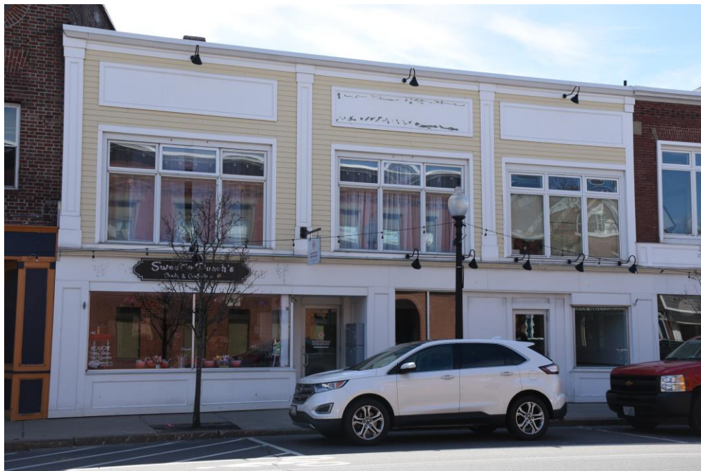
Photo 36) 16-22 North Main Street, looking southwest
