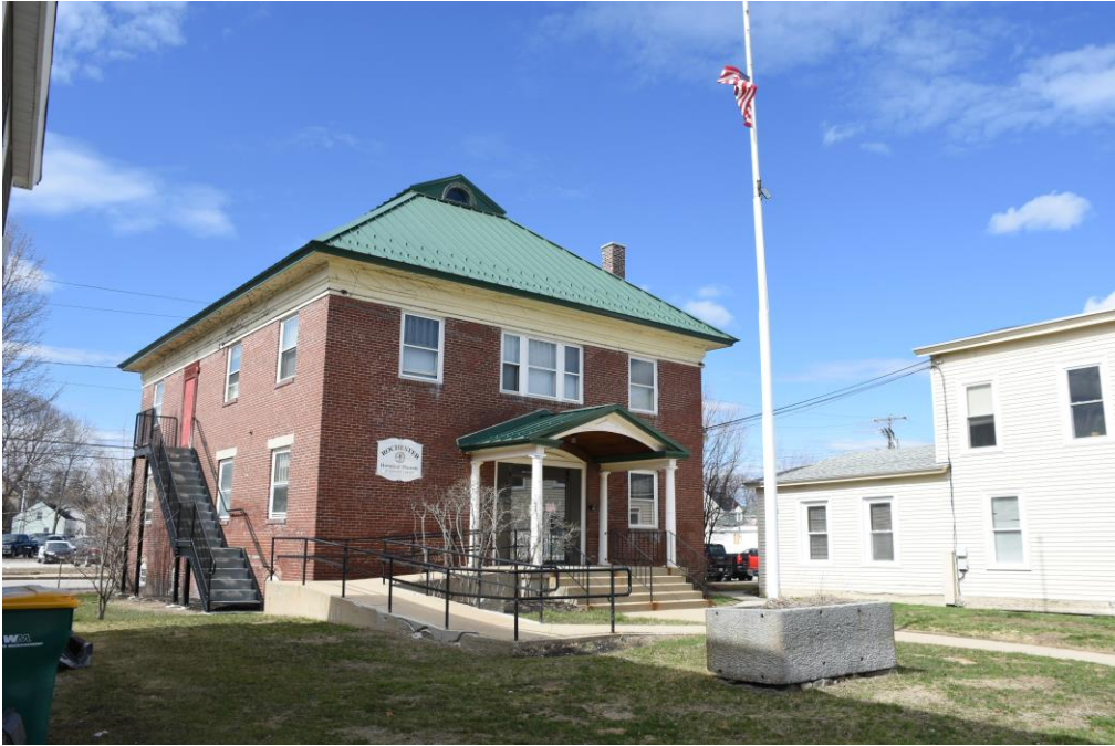
Photo 80) 58 Hanson Street, looking north
