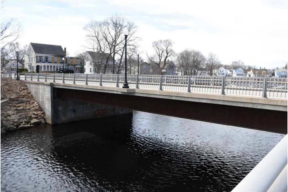
Photo 68) Bridge Street Bridge, looking west
