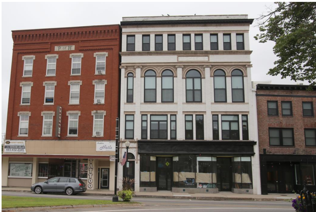
Photo 34) 10 North Main Street, looking southwest
