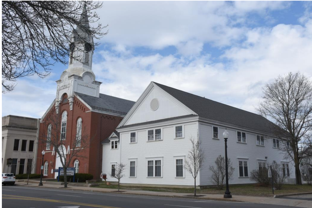
Photo 87) 34 (left) and 36 (right) South Main Street, looking northeast
