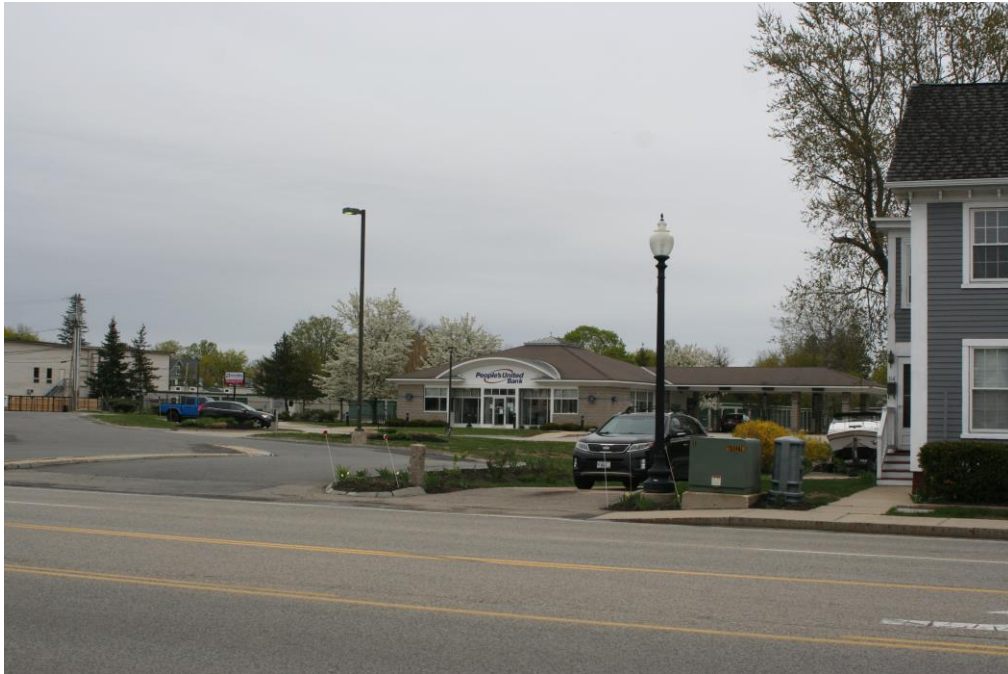
Photo 107) 110 South Main Street, site of former Wallace Shoe Factory, looking northeast
