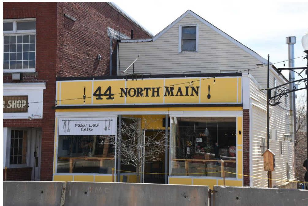
Photo 42) 44 North Main Street, looking south
