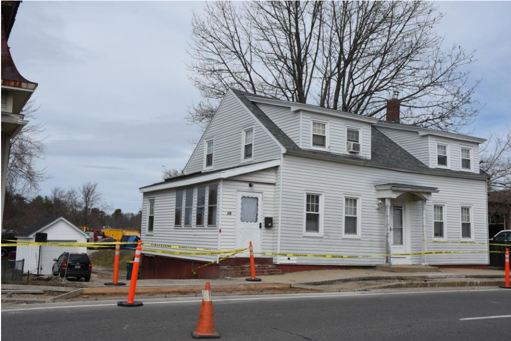
Photo 62) 16 Union Street, looking north
