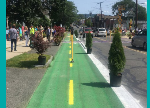
Temporary bike lane
