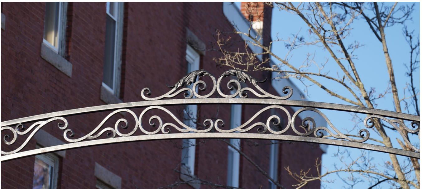
Figure 74. Arch above Factory Court Pedestrian Walkway
